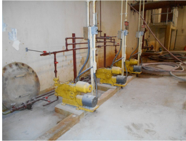
FIGURE 3-40 POLYMER PUMPS
