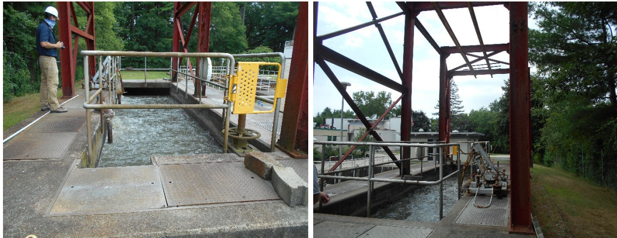
FIGURE 3-8 AERATED GRIT REMOVAL CHAMBER
