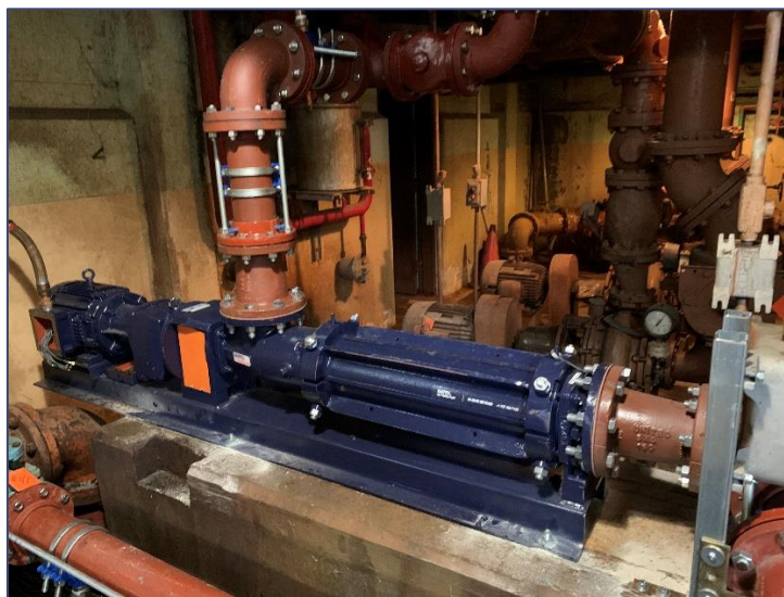
New DSTP #1 Install
