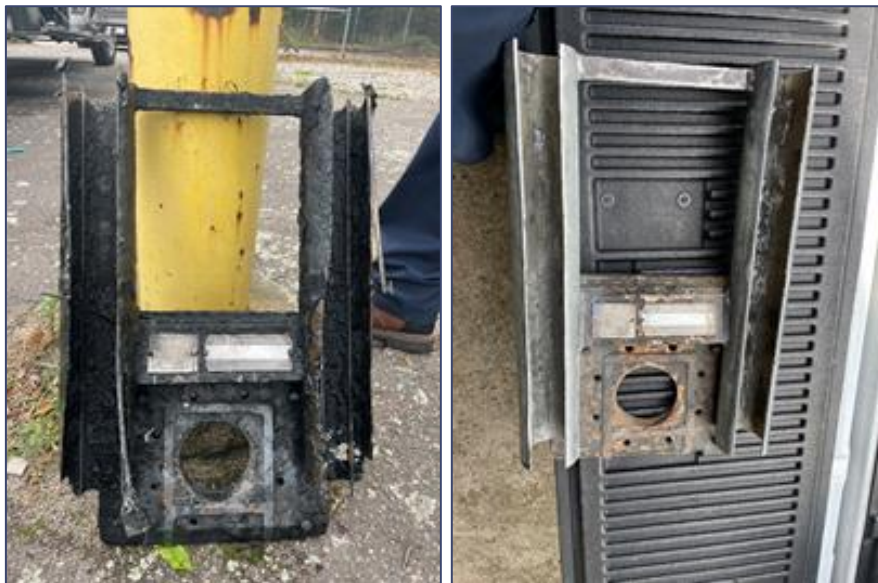
OCW Pump Bracket Before and After
