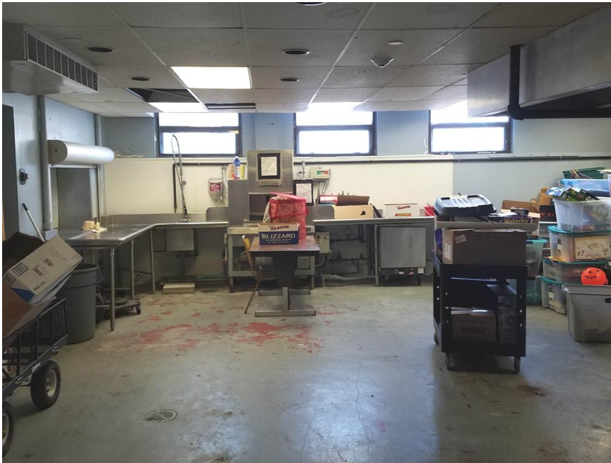
Decommissioned Kitchen/ Storage
