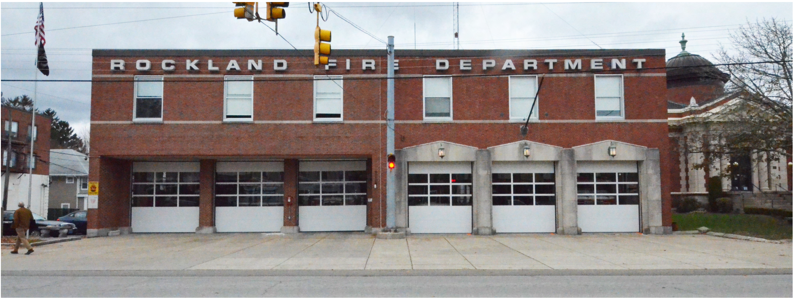
Existing Fire Department Headquarters 360 Union St, Rockland MA
