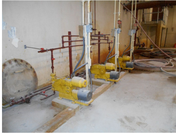
FIGURE 3-40 POLYMER PUMPS
