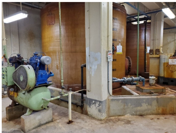
FIGURE 3-35 AIR COMPRESSOR
