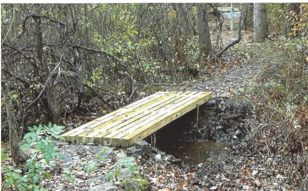
A new design for trail bridges in wetlands made to last.
