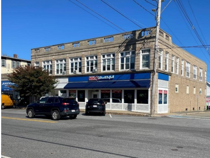
Figure 3: Existing Facade on Union Street
