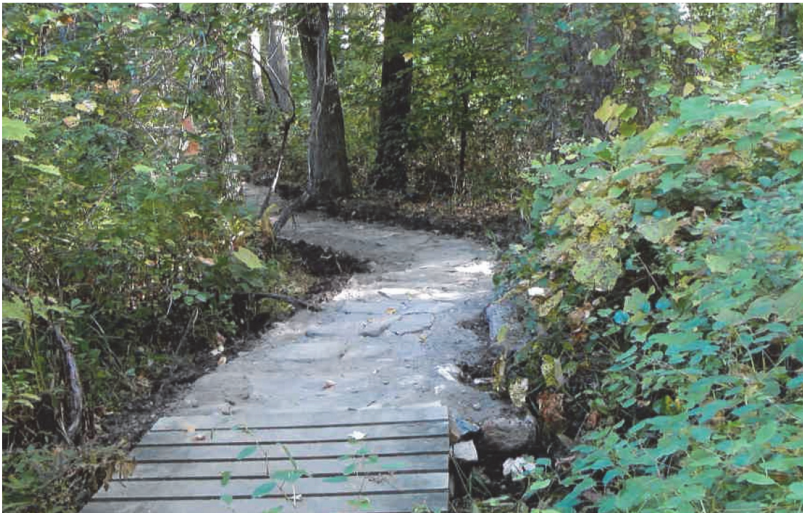
This photo shows a portion of the trail improvements made in 2020.
